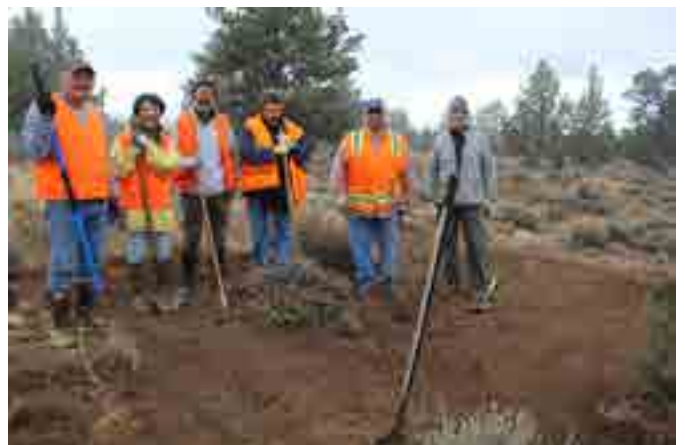
Crew after filling and leveling dig site.
