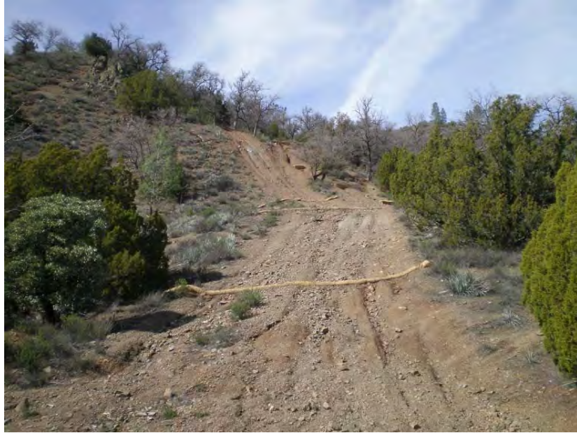
Figure 4. OHV impacts and erosion on Gaviota soil series (above Jade Mill campground) within the CCMA. Erosion control including straw bales and straw rolls were installed in gullies and rills to slow erosion.
