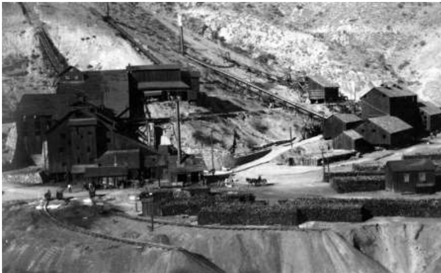
Figure 5. New Idria mine circa 1910. Stacks of cord wood (foreground) obtained from within the CCMA to fuel the cinnabar retorts.
